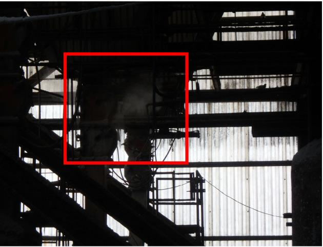
• Baghouse fly ash leaks at either the dual flap valve or the hopper.
